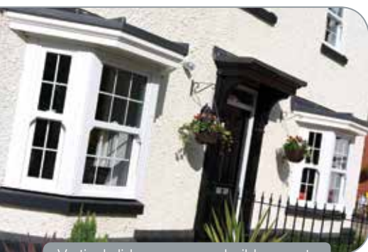
Vertical sliders on a new build property
